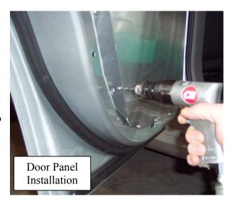
Note: apply wax to screws to avoid screw head from snapping.
